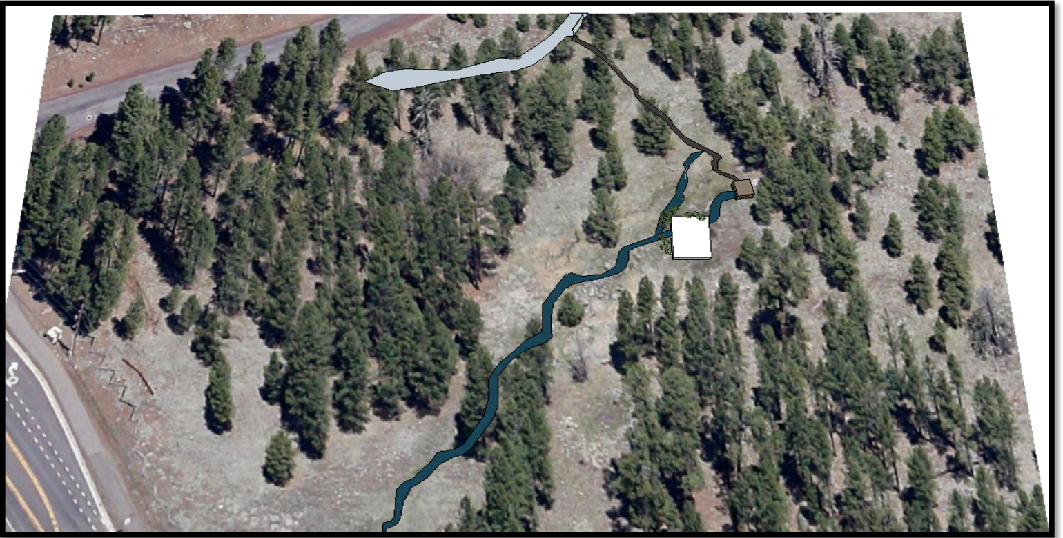
Figure 12- The current site location with the concrete box
