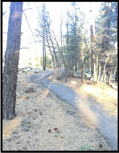
Figure 4- Non ADA compliant section
