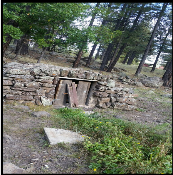
Figure 6- spring box flow in fall 2015 with door
